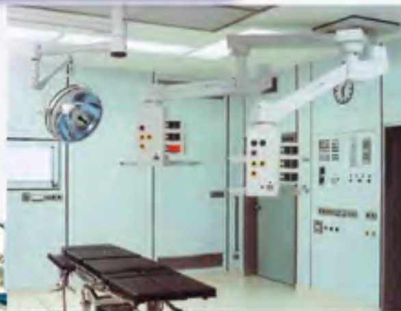
Franke bearing elements in a medical ceiling system. Easy manual swivelling movements in spite of heavy loads.
